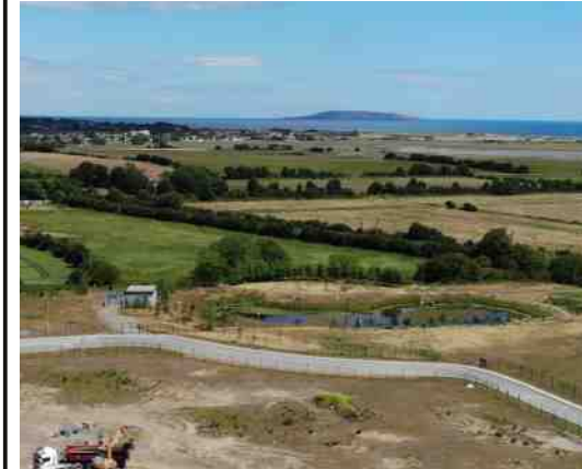
Attenuation pond and Wetland Park under construction
