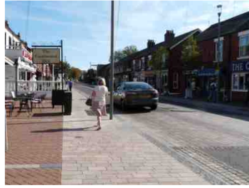
Flush surfaces encourage driver caution
