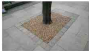
Resin Bond Tree Pit'
